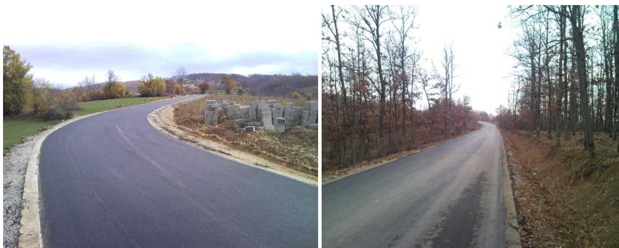
Ndërtimi i rrugës Mohlan- Krushicë
